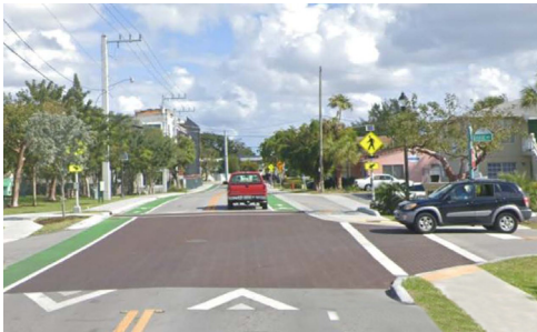
An example of a raised intersection similar to Riverland Road at a sidestreet
