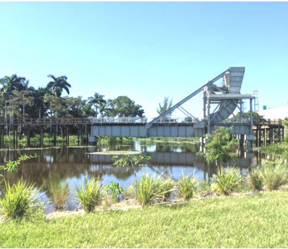
The 1926 CSX Railroad Bridge
