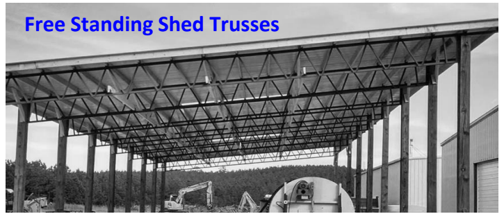
Bar Joist-Header Truss
