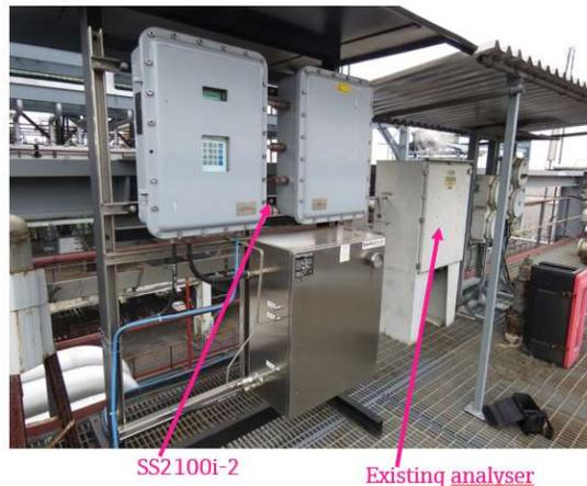
Fig: 1. TDL analyser and the existing analysers as installed at site.
