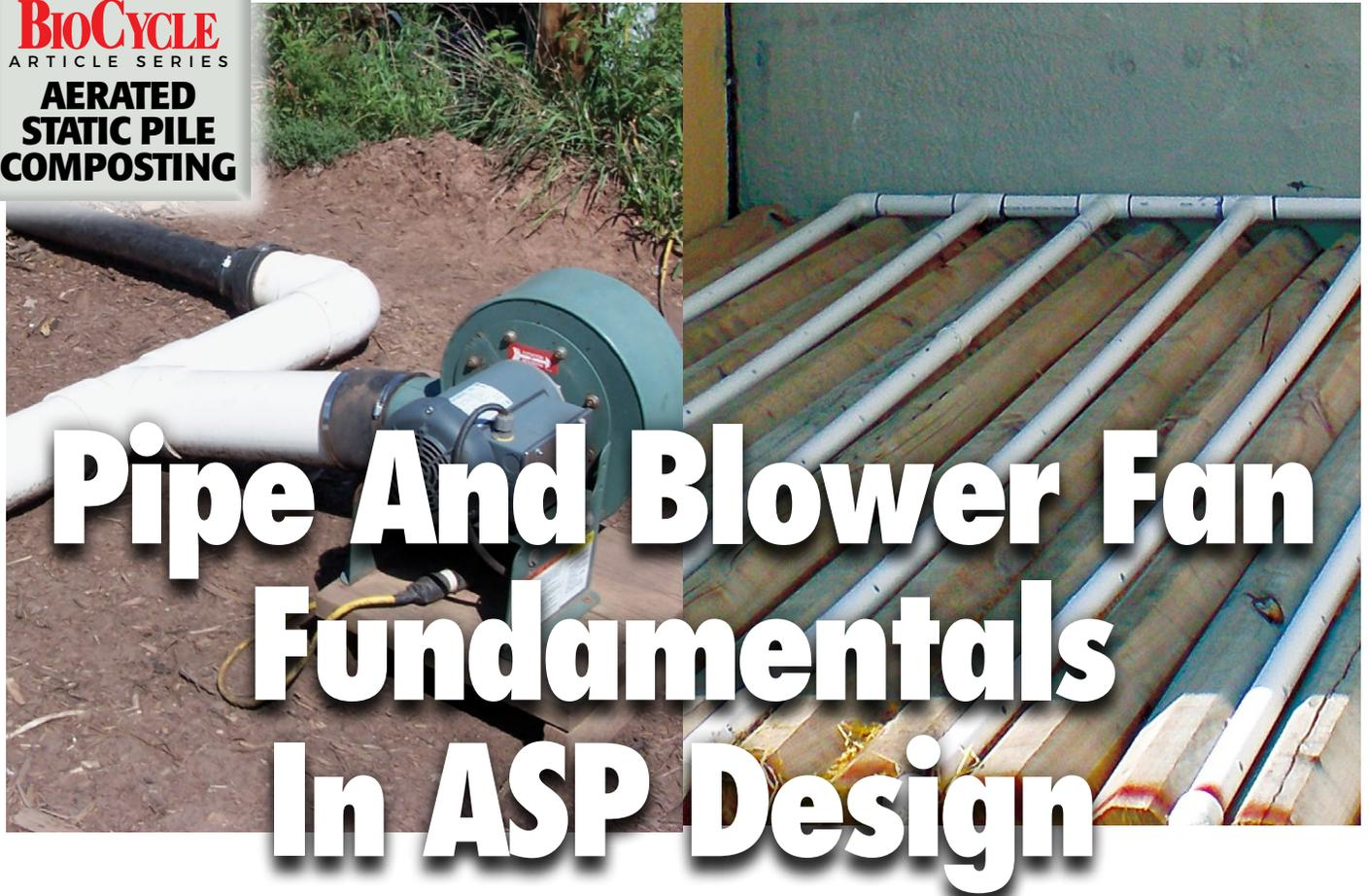
**ASP composting designs most often use centrifugal blowers (left), as these are recommended for systems with back pressure caused by having long runs of piping or ducting. Facilities can test various piping system designs, such as entrenching the pipes as shown in this pilot test (right).**
