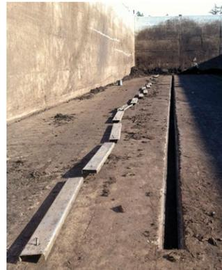
**Figure 3. Trench covers removed for maintenance**
