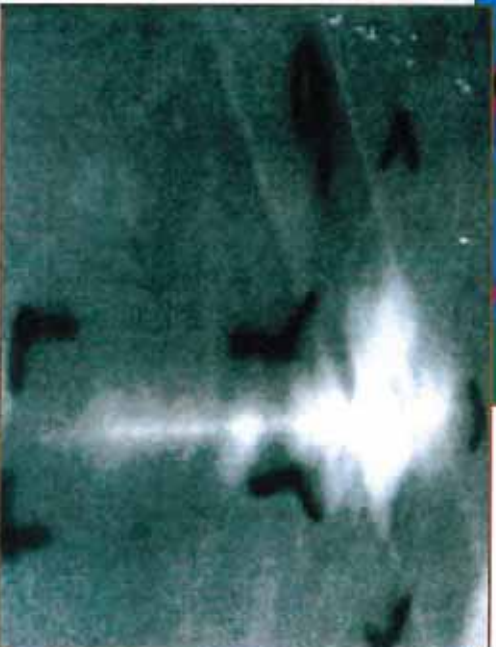
Photograph 4: View of wet insulation occurring along joint between ISO boards (gray contrast).
