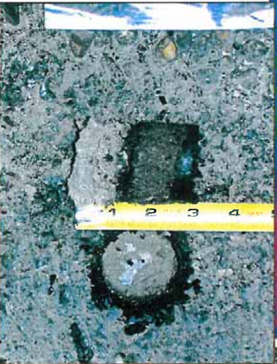
Photo 22 – Core showing wet upper layer of perlite in BUR.
