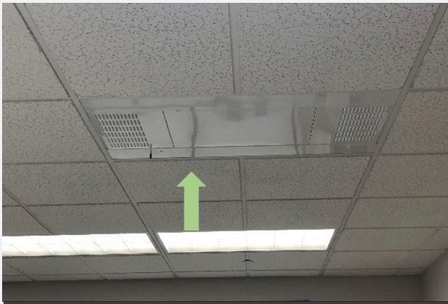
BOA Vista Towers office space installation
