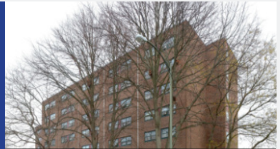
Boa Vista Tower's High-Rise Building
