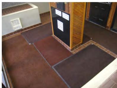
Quarry tile floor at entrance vestibule nearly completely covered with walk-off floor mats.
