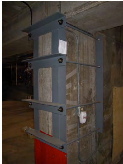
Cast-in-place concrete column reinforced with steel angles and tie rods.
