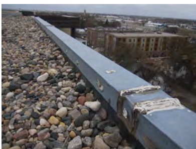
Original flashing at the 9 th Floor Roof.
