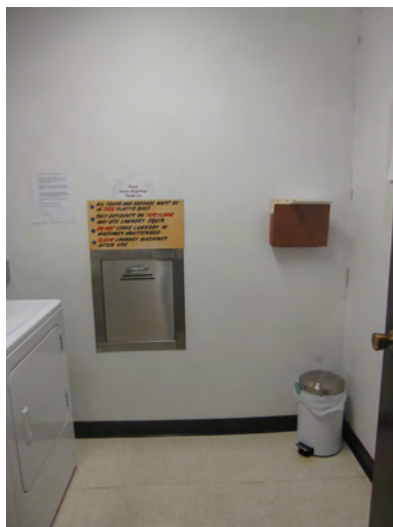
Typical trash chute.
