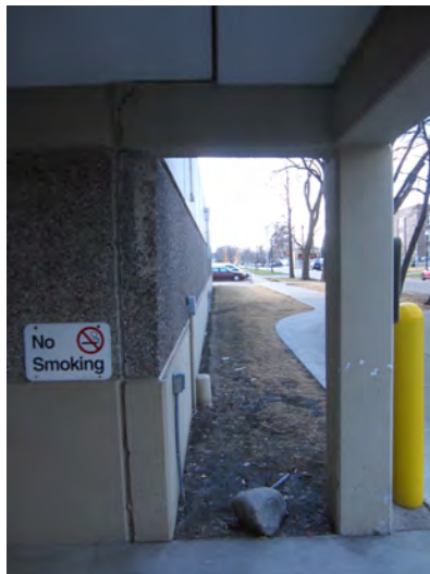
Precast column and beam on the west side of the north entrance.
