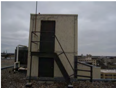
Wood guardrail at the bottom of the ship's ladder.
