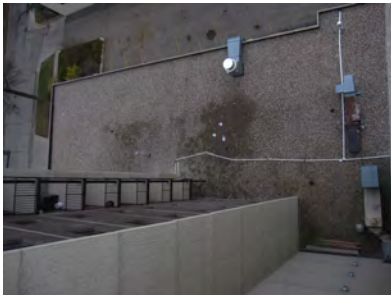
Southeast corner of the garage roof.
