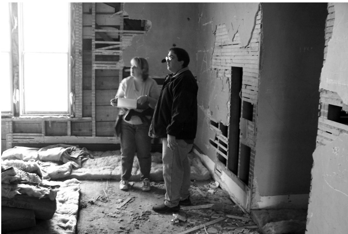
Figure 5: Wall 5 behind Jason, Wall 6 behind Vi.
