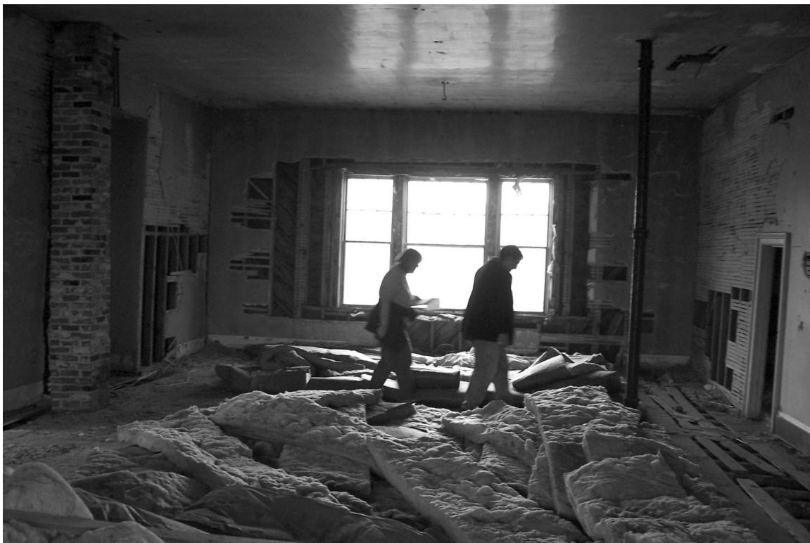
Figure 6: View of East End of Room – Walls 6-7 in background.
