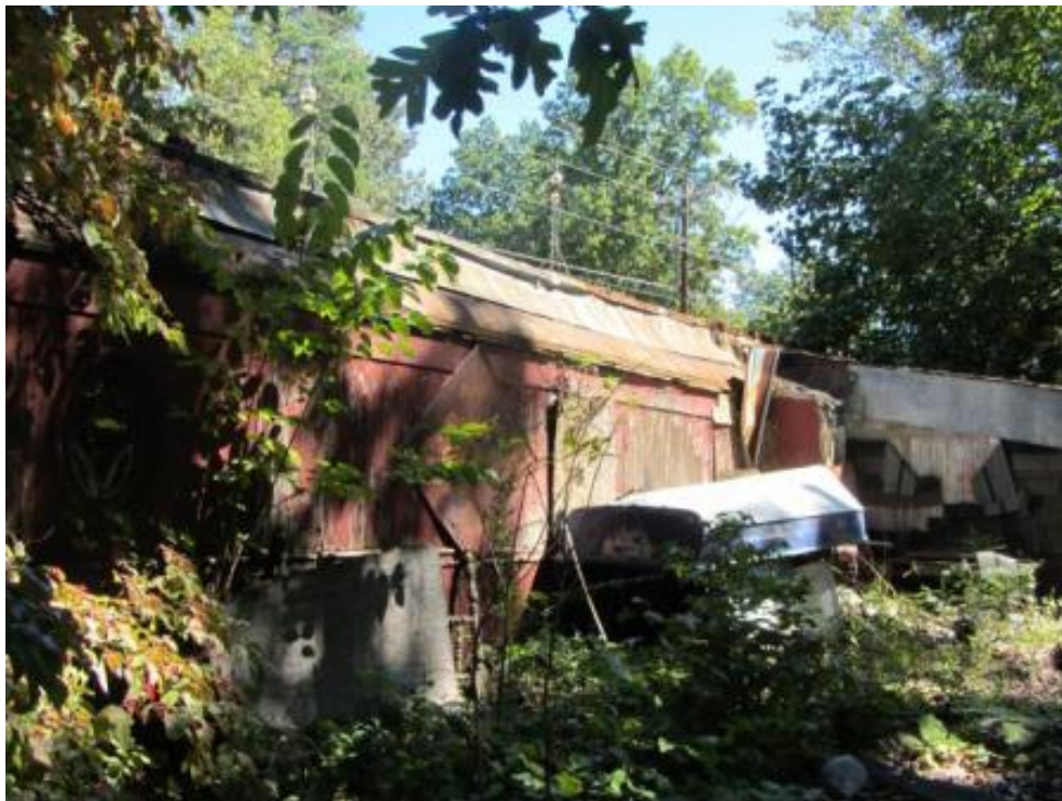
Figure 33. NCDOT Survey #33, Midway Diner (GF-1545), 6270 Burlington Road, Guilford County, south elevation of diner with a section of kitchen addition visible, looking northeast from driveway.
