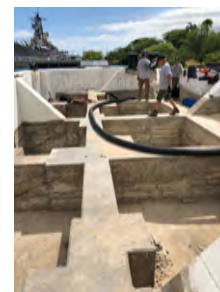
Exposed structure after sand removal
