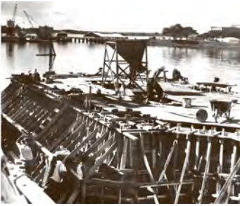
Fleet Mooring historic construction photo
