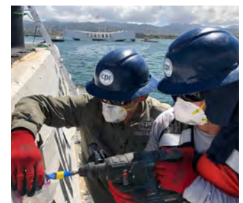
Concrete drilling to collect samples for chloride testing
