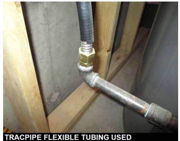
TRACPIPE FLEXIBLE TUBING USED
