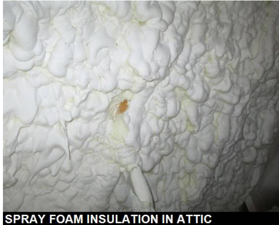
SPRAY FOAM INSULATION IN ATTIC
