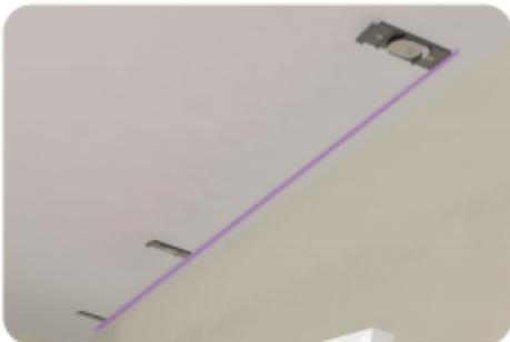
The most difficult part about installing traverse rods is getting the brackets even, level, and straight. A variance of as little as a 1/8" can prevent you from being able to install your rod correctly. Choose your desired location to mount brackets and mark with a pencil. Make sure that all brackets are aligned evenly across and verify using a level. Brackets should be positioned every 3-4 FT. Never, under any circumstances, use hollow anchors with brackets.
