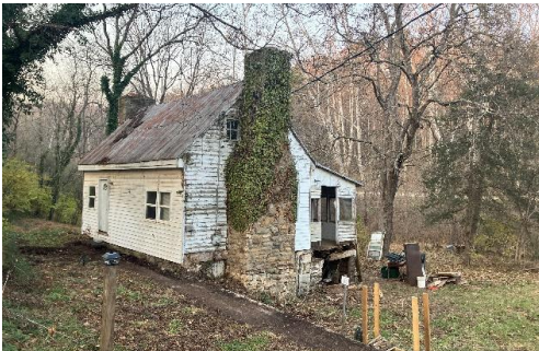
The cabin after bush hogging and removing the deck and steps.
