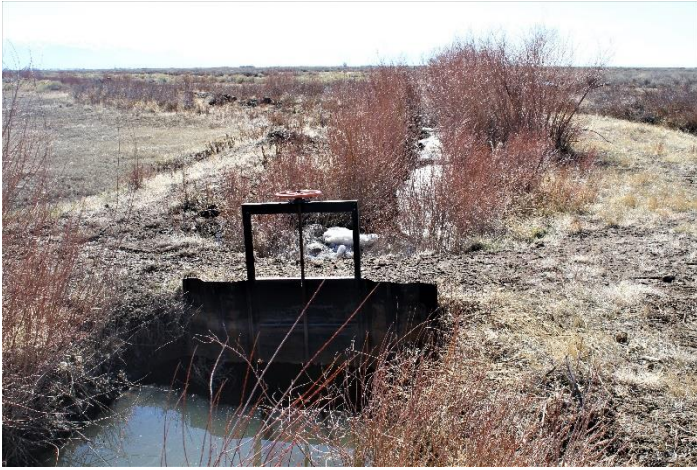
Headgate looking downstream
