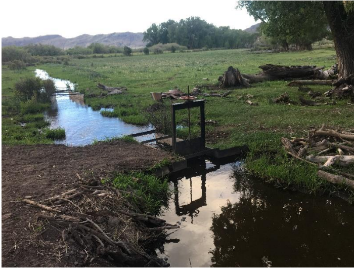
Headgate looking downstream
