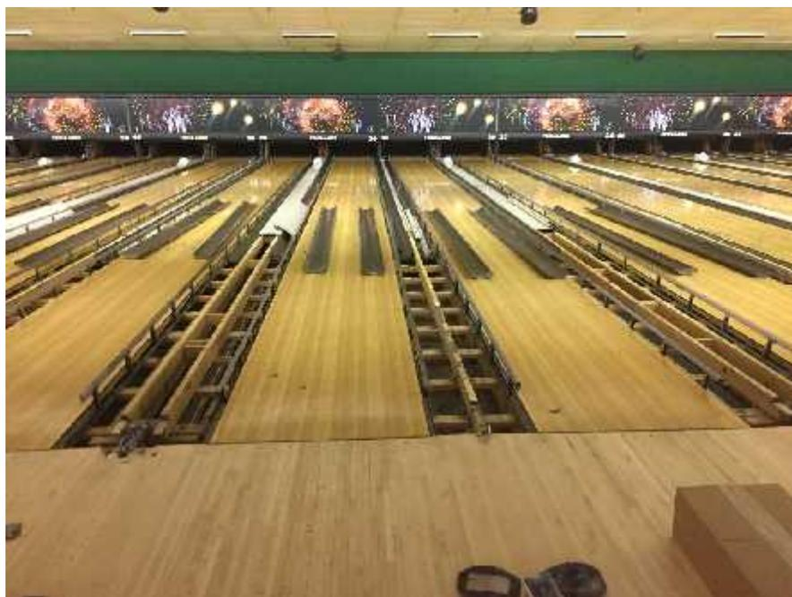
We ran the Home Run line to the Control Desk from Lane 1 for Auto-Bumper Control, and wired the 5 Power Supplies in 8-lane groups across the curtain wall. We programmed the BCU II addresses into the Bumper Controller (shown below at the control desk).
