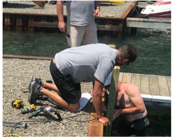
Installing new uprights on new seawall!
