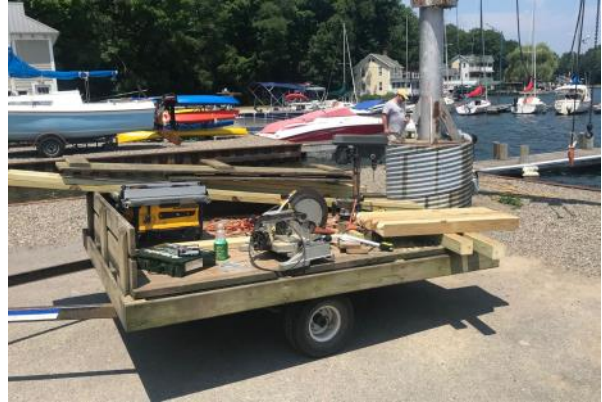
Gearing up for repair work!
