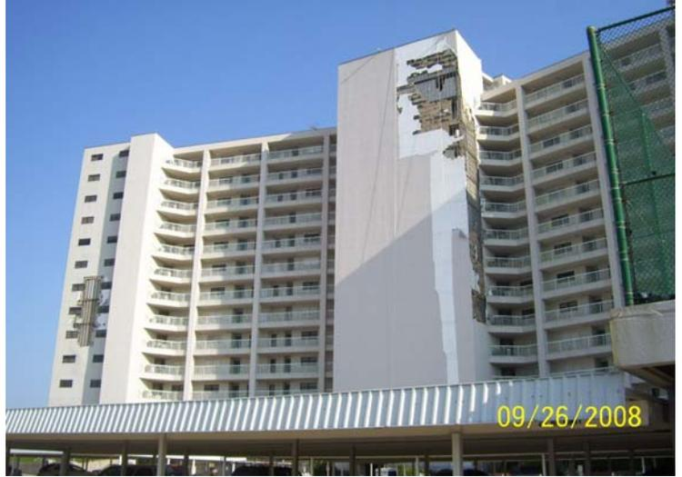
The Breakers is a 13-story steel-framed high-rise condominium that was constructed in 1983 and located on Seawall Boulevard with ocean-front view in Galveston, Texas. In 2008, Hurricane Ike caused physical damage to the existing EIFS on the exterior walls of the North elevation of the building. The exterior wall construction consisted of a EIFS over exterior-grade gypsum sheathing over light-gauge metal studs with painted interior gypsum sheathing.
