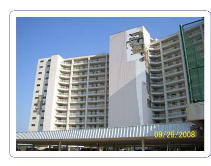
The Breakers is a 13-story steel-framed high-rise condominium that was constructed in 1983 and located on Seawall Boulevard with ocean-front view in Galveston, Texas. In 2008, Hurricane Ike caused physical damage to the existing EIFS on the exterior walls of the North elevation of the building. The exterior wall construction consisted of a EIFS over exterior-grade gypsum sheathing over light-gauge metal studs with painted interior gypsum sheathing.
