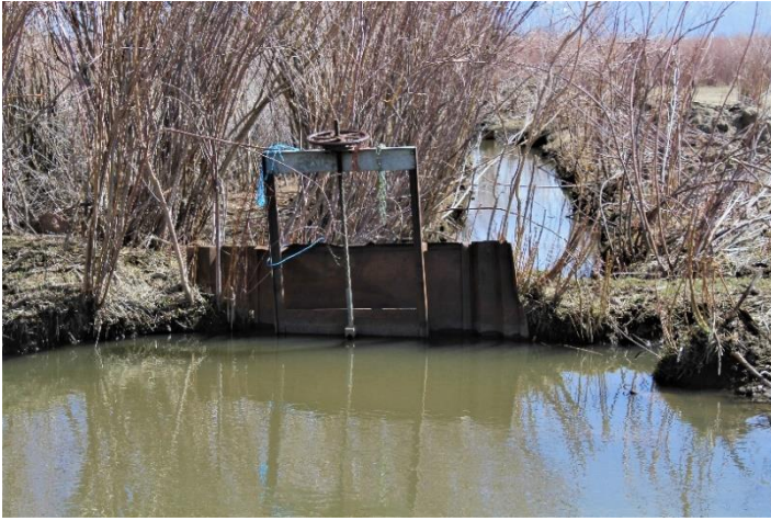
Headgate looking downstream
