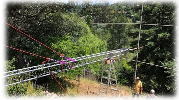
The lowering took place by removing a pin at the rear of the base to release the tower for pivoting. The weight of the tower was now supported by the pivot at the base and by the lowering rope from above. Once the tower had cleared a roof obstruction, it was lowered toward a ladder set up to support the tower for disassembly.
