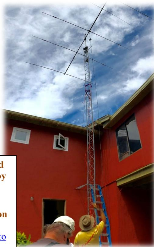
Jay created a pulley system to lower the tower. The lowering rope used a pulley at the edge of the roof. Another rope was attached to the chimney to provide guidance and support. That rope could also be used to re-raise the tower if
