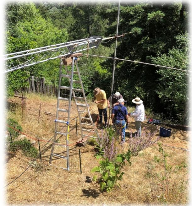
The disassembly of the antenna sections required a series of rotations and section removals. Ultimately the entire antenna mast and rotor were removed prior to disassembling the tower itself. The tower was disassembled from the bottom section to the top, section by section. The remainder of the tower was slid toward the house as each section was removed.
