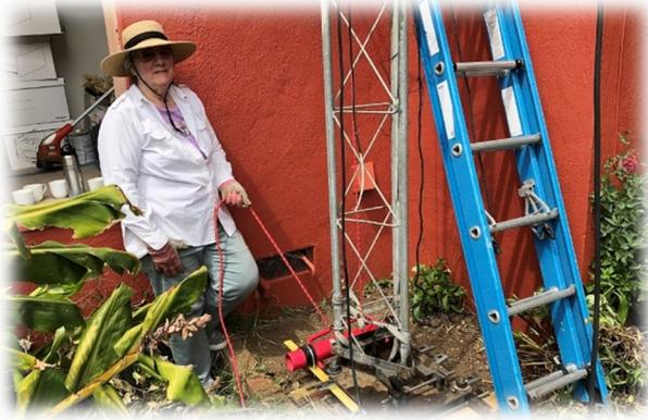
necessary. An additional rope extended downward and enabled the tower to move laterally, if required, to guide its descent. The lowering rope supported the entire weight of the tower as it descended.
