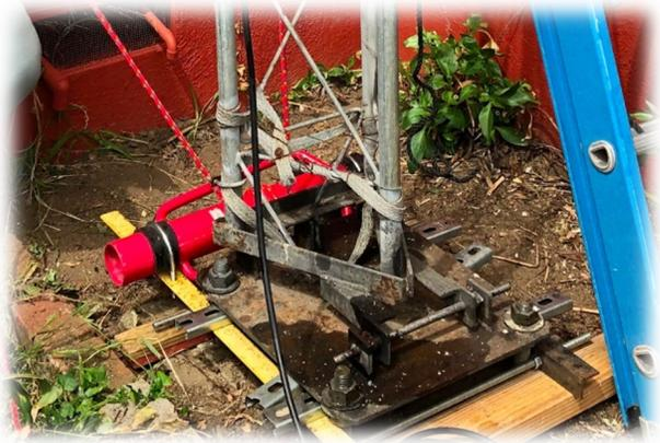
(mounted with four bolts to the concrete footing) and a triangular steel structure at the bottom of the tower. This piece was attached to the steel base with a pivot pin. The tower was mounted in a pivoting base that would allow it to be lowered intact and disassembled. The antenna spanned 23 feet and was mounted on a rotor. The tower, with its bottom three sections, extension on its topmost section, additional steel plates, and antenna section weighed approximately 200-225 lbs.
