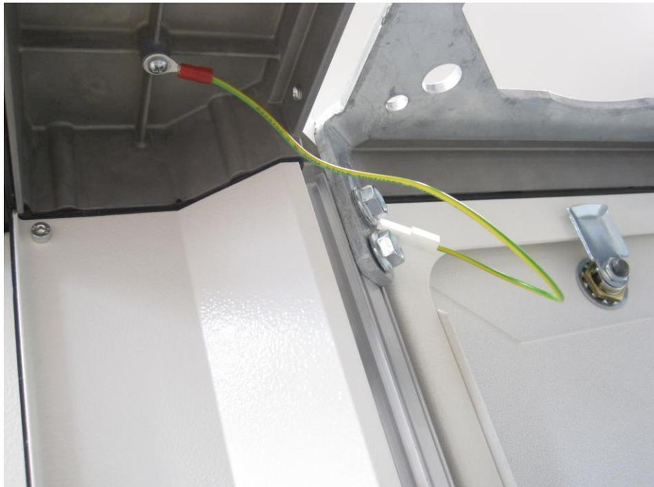
*Drawing 27 - Intermediate hood earthing connection*
