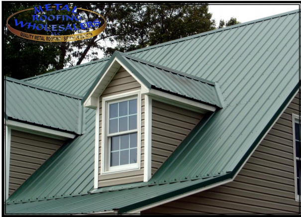
Figure 1 House With Classic Rib® Metal Roofing Installed
