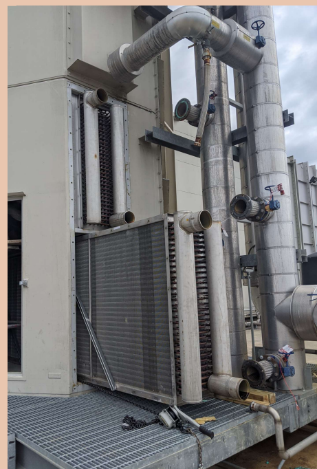
Safe Module Removal
