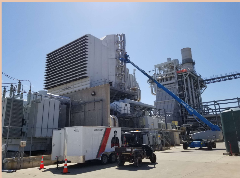
Complete Turn-Key Chiller Repair & Cleaning
