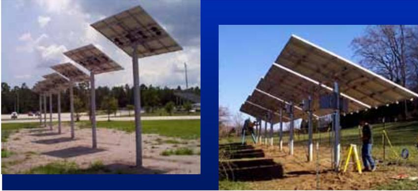
Figure 23. Pole-mounted arrays use either fixed, adjustable, or sun-tracking arrays installed on a rigid metal pipe.
