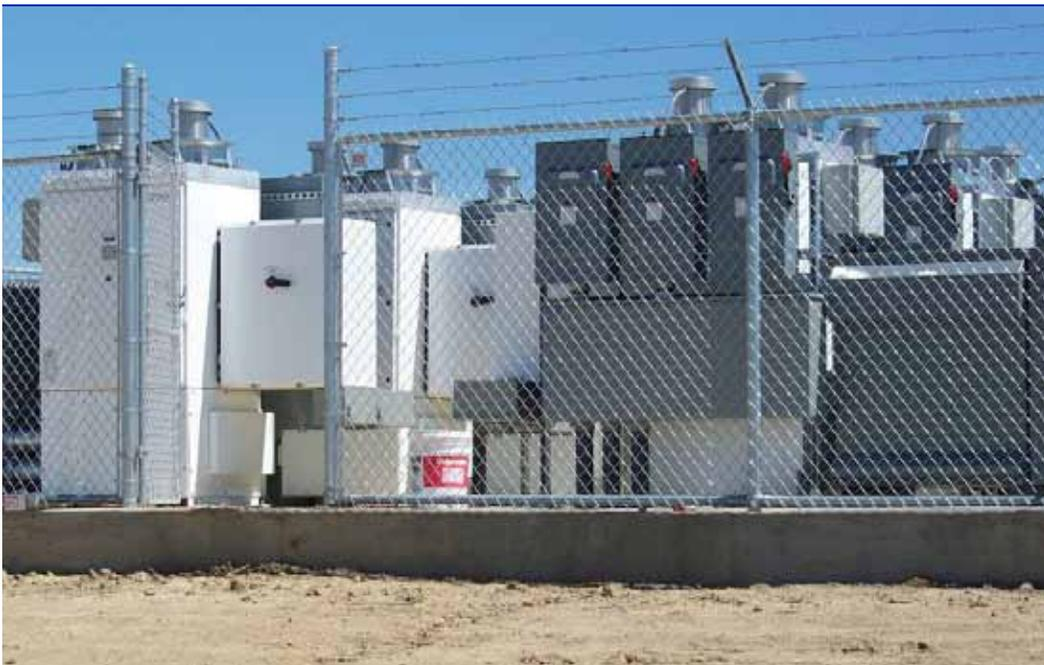
Figure 74. Utility-scale inverters use higher DC input and AC output voltages to reduce losses, and the size and costs of the conductors and switchgear required.
