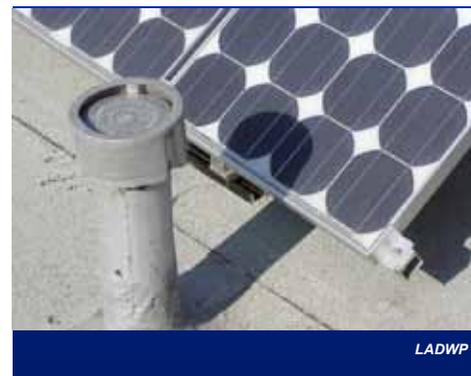
Figure 17. Shading of PV arrays can be caused by any obstructions interfering with the solar window.
