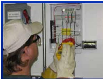
Figure 111. Operating parameters in PV systems are measured to verify expected performance.
