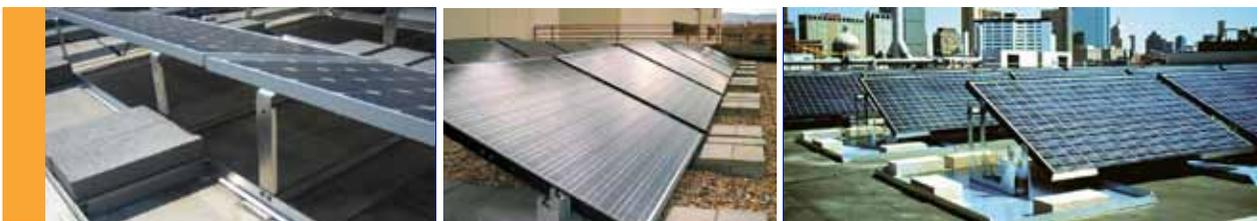
Figure 22. Self-ballasted PV arrays are a type of rack mount that relies on the weight of the PV modules, support structure and additional ballast material to secure the array.
