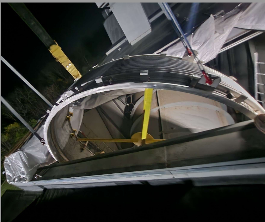
Turn-Key V84 Outlet Bellows Replacement
