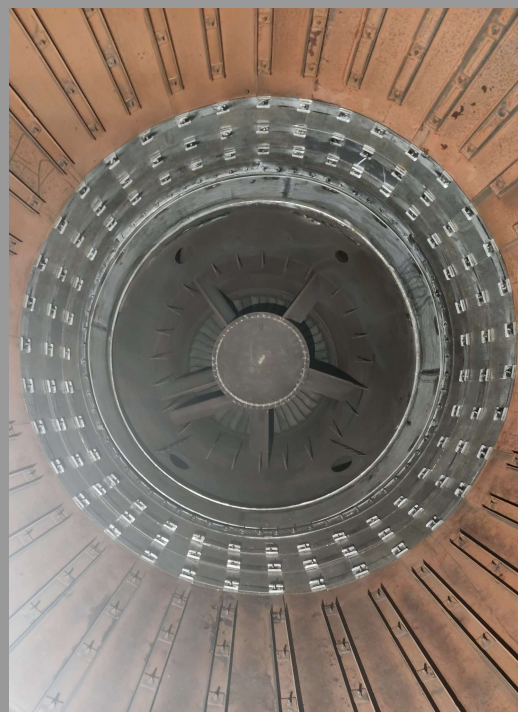
Liner System Over Transition Immediately Downstream of Bellows
