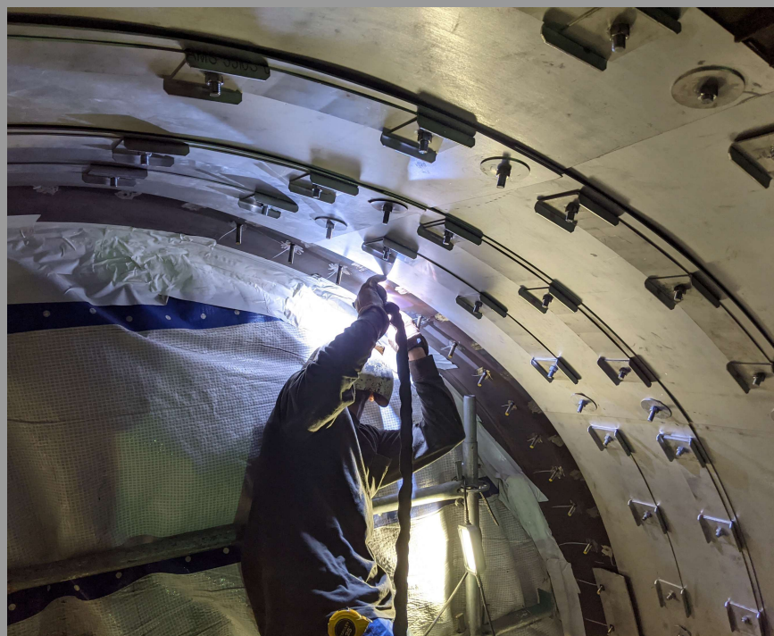
Liner System Over Transition Immediately Downstream of Bellows
