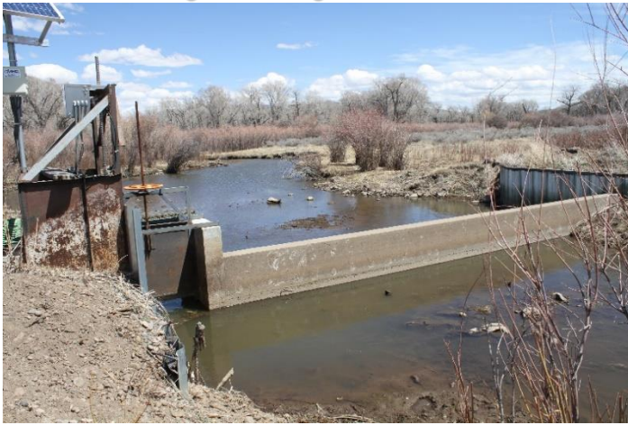
Headgate looking downstream
