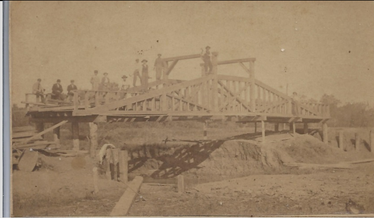
A Bridge Under Construction
