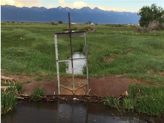
Headgate looking downstream
