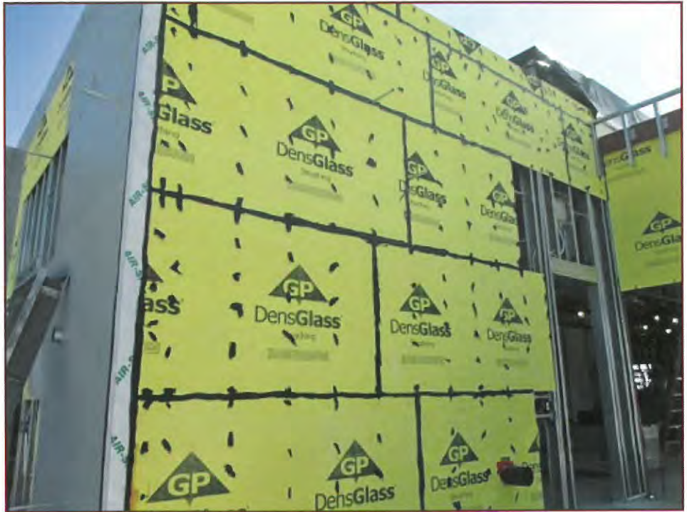
Figure 3 – Pretreatment of sheathing joints and fastener heads.
