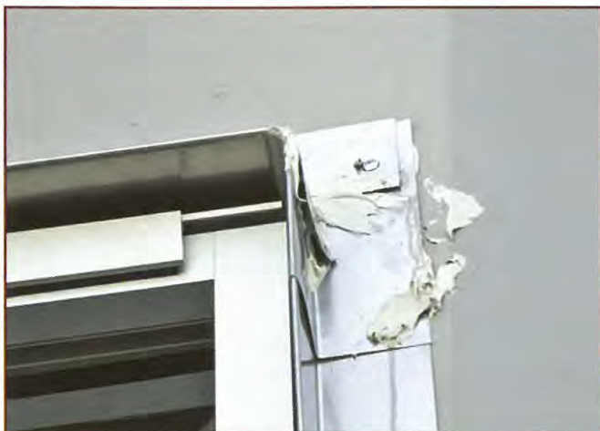
Figure 13 – Corner joint of sheet metal flange installed around window opening.
