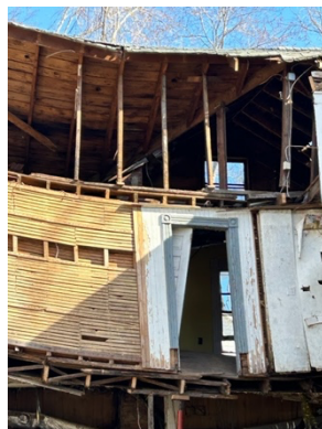
Shored Up Walls
