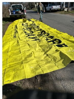
Tarp for Roof
