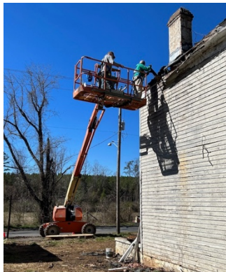
Cutting Off the Rotten Roof
