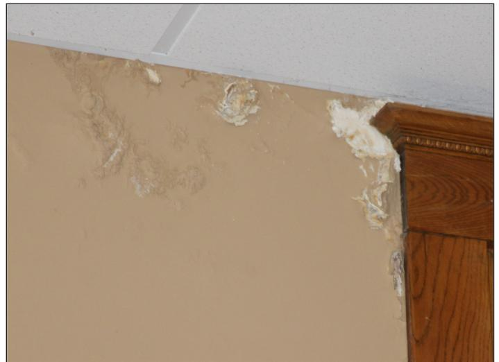
**INTERIOR DAMAGE TO THE CARNEGIE RESOURCE CENTER IS EXTENSIVE. Clockwise from above left: The east wall of the gallery has damaged plaster and water pooling behind the paint; Water has also pooled behind paint on the west wall of the gallery room; Paint and plaster have been flaking off the walls of the Weller Room; The northwest corner of the West Room has been severely damaged by water leaking through.**
