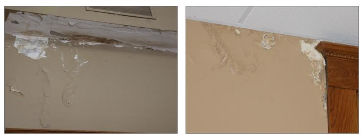
INTERIOR DAMAGE TO THE CARNEGIE RESOURCE CENTER IS EXTENSIVE. Clockwise from above left: The east wall of the gallery has damaged plaster and water pooling behind the paint; Water has also pooled behind paint on the west wall of the gallery room; Paint and plaster have been flaking off the walls of the Weller Room; The northwest corner of the West Room has been severely damaged by water leaking through. See more photos of damage on page 15.
