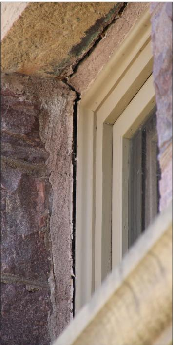
WATER REALLY AFFECTED THE CARNEGIE RESOURCE CENTER IN MITCHELL THIS YEAR. Clockwise, from left: Water damaged the stone on the outside of this window ledge on the south side of the file room; The stone has been damaged on the northwest corner at the entrance of the building; Many walls inside the building have been heavily damagd by water, especially the northwest corner of the west room; the windows are separating from the stone on the northside of the main entrance to the building.
