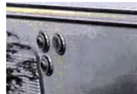
Another option would be to drill 2 new 2 ¼" holes and leave the original holes capped off. This would leave the exterior looking like:
