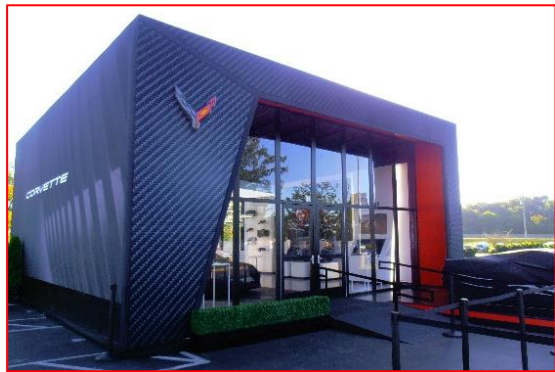
This temp structure was put up overnight & showcased C8 wheel, colour & seat samples.
