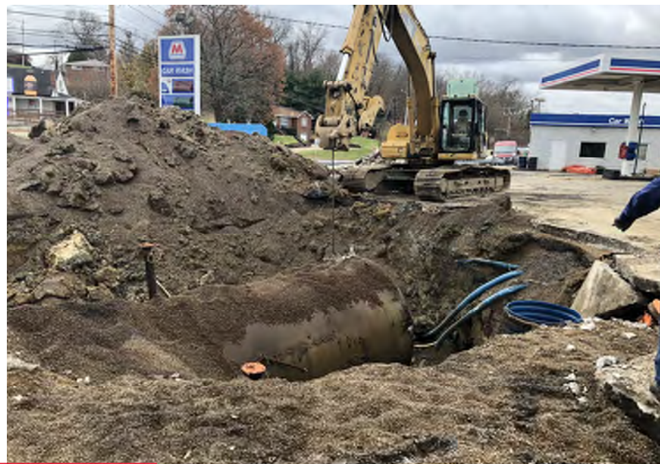
Gas Tank-3 Removal
