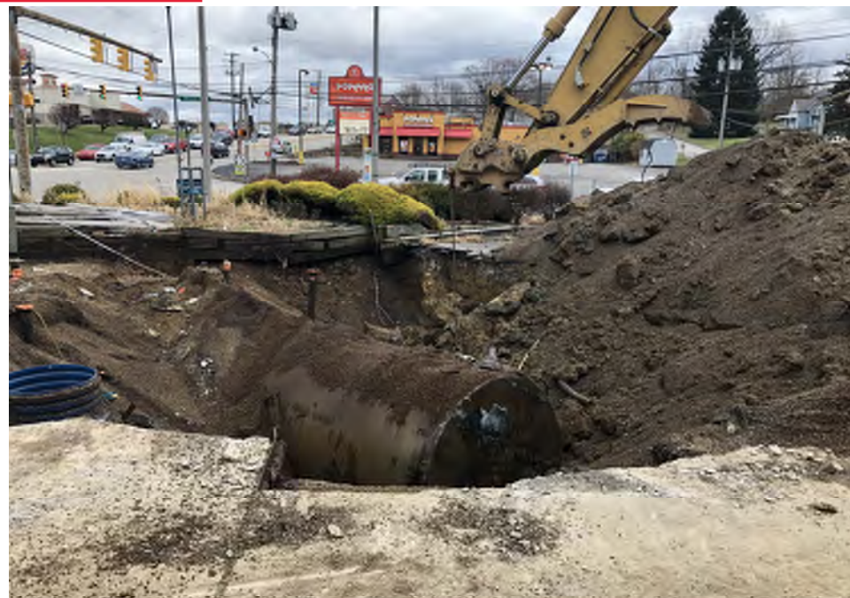
Gas Tank-3 Removal
