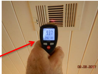
The furnace in the attic was sealed and was not accessible to inspect the heat strips. The output at the diffusers is indicating normal operation in the heat mode.
