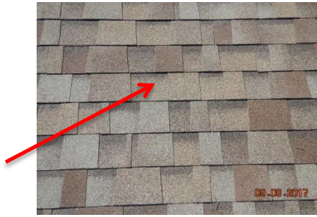
The roof covering is a laminated 30-year roof covering.
