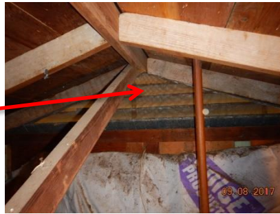
The attic is ventilated by gable vents.
