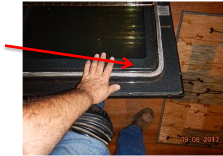
The range is not connected to an anti-tip device.
