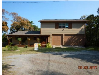
South side of the home.
