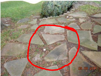
The current home owner says the septic tank is below this rock.
