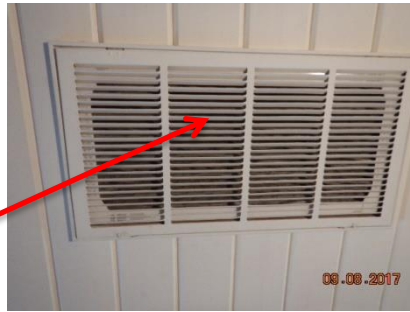
The HVAC return filter is in the den ceiling and is a 12" x 24" x 1" disposable filter.
