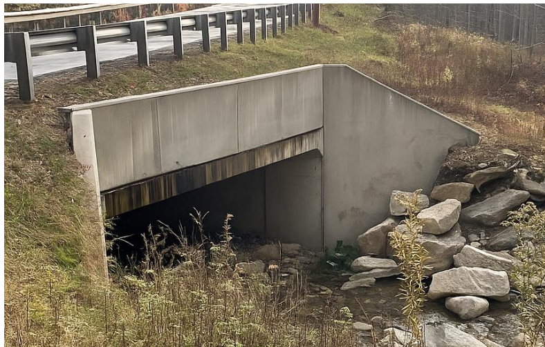
Top photo: Kidder Brook culvert washout during Tropical Storm Irene, 2011 Bottom photo: Enlarged structure installed following TS Irene
