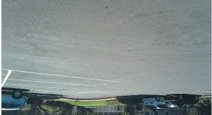
This component is for seal coating and striping of all asphalt. Asphalt should be seal coated every 5 yrs to protect the base surface from the destructive UV ray. New Asphalt should be seal coated with in the first 2-3 years to protect the base coat.
