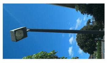
The street lights are very energy inefficient. Recommend replacement with solar LED lighting for energy saving. Current light fixtures are decaying rapidly and nearing their useful life.
