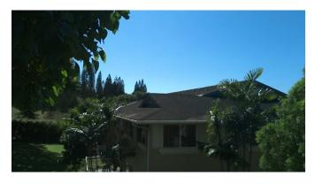
There are approximately 1400 squares of asphalt shingle of roofing. The current roof appears to be a 20-30 yr roof, however according to management roof inspections have reported that it will not last more than another few years. Recommend replacement with at least a 30 year roof.
