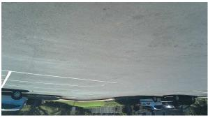
This component is for seal coating and striping of all asphalt. Asphalt should be seal coated every 5 yrs to protect the base surface from the destructive UV ray. New Asphalt should be seal coated with in the first 2-3 years to protect the base coat.
