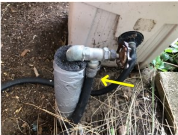
Exterior hose spigot(s) do not have code approved anti-back flow devices installed.
