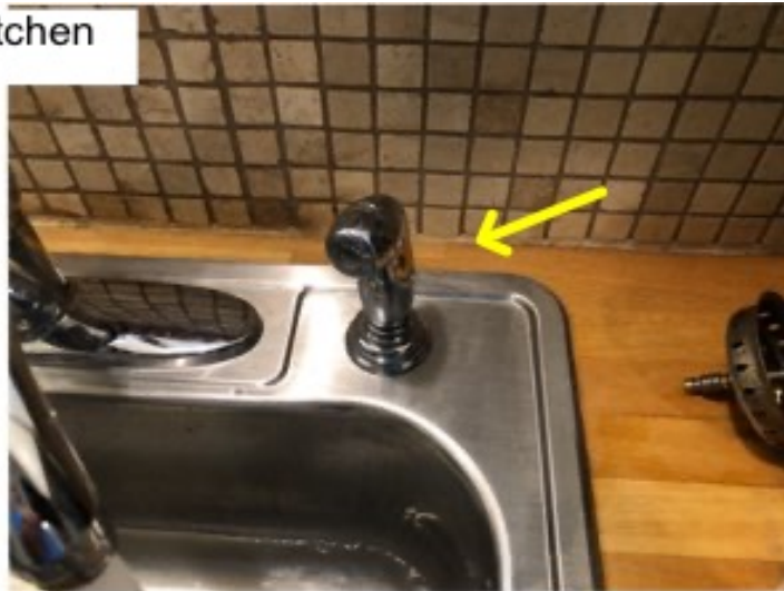
Kitchen sink spray wand not functioning
