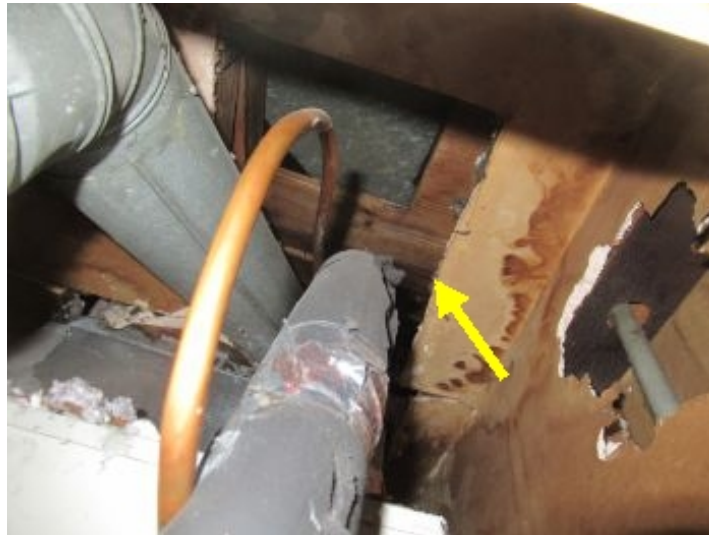
Ceiling above air handler is open allowing for debris to enter mechanical closet
