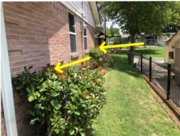
Bushes / trees / foliage should not contact siding of building to prevent damage and insect access
