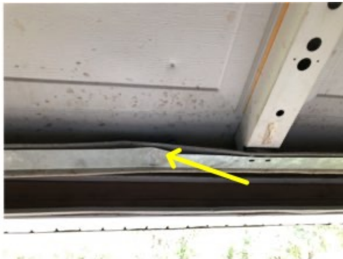
Garage door is damaged/bent
