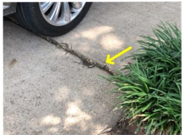
Driveway has settled and has multiple cracks and uneven surface.
