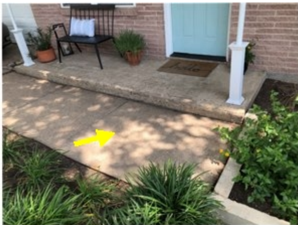
Sidewalk slopes towards front porch
