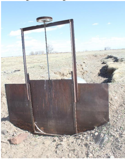
Headgate looking downstream
