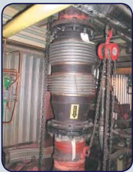
Universal Exp Joint for Process
