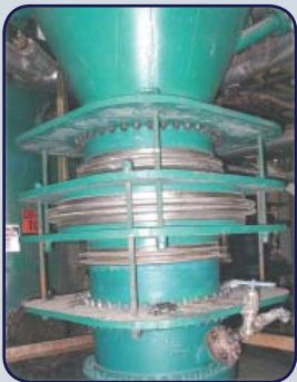
In-Line Pressure Exp. Joint
