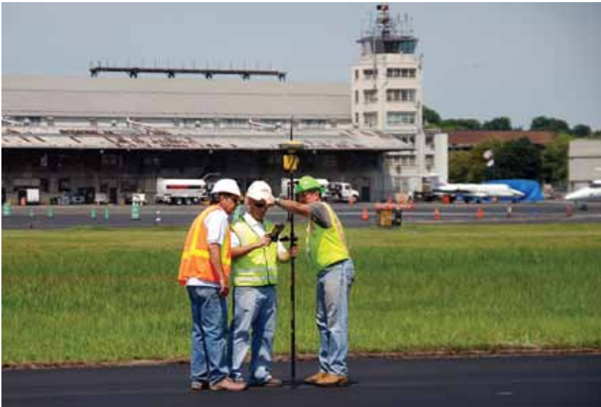
Surveyor Jamie Lovaglio and Super John Carollo are checking finished grades with Topcon dealer Jim Cleary.
