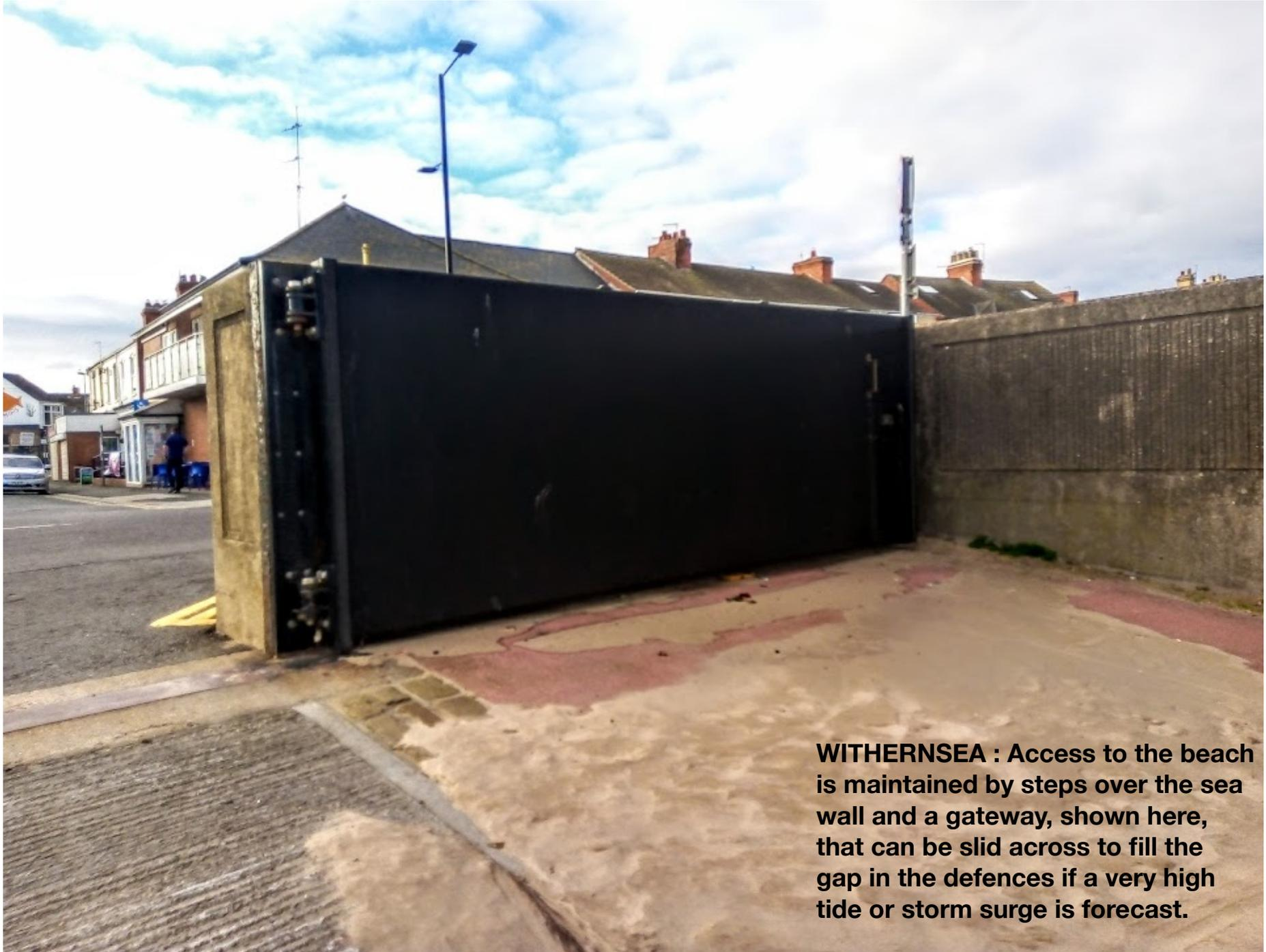
**WITHERNSEA : Access to the beach is maintained by steps over the sea wall and a gateway, shown here, that can be slid across to fill the gap in the defences if a very high tide or storm surge is forecast.**
