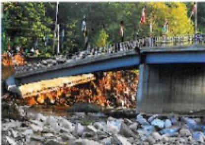
**Loon Mountain Bridge (Lincoln, N.H.) collapsed due to heavy scouring around the abutment after 11" of rain.**
