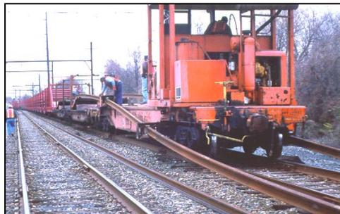
This project provided for the installation of new 115# continuous welded rail on Track # 1 from Manayunk Station to 16<sup>th</sup> Street Junction and Track #2 from 16<sup>th</sup> Street Junction to Scotts Lane in Fiscal Year 1999. In Fiscal Year 2000, this project provided for the installation of rail on Track No. 2 from Scotts Lane to River Crossover. This project reached completion in June 2000.
