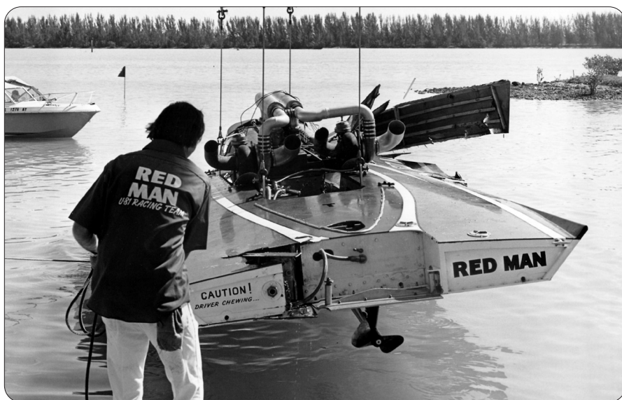
TOP: Skipp Walther settles into the cockpit of the U-81 Red Man before heading out onto Biscayne Bay at Miami in 1974. MIDDLE: The Red Man is hoisted from the water after the accident that killed Walther. The boat's right sponson was extensively damaged when the boat spun out. ABOVE: The rear of the Red Man after the accident in Miami. Note that the rudder is completely missing.
