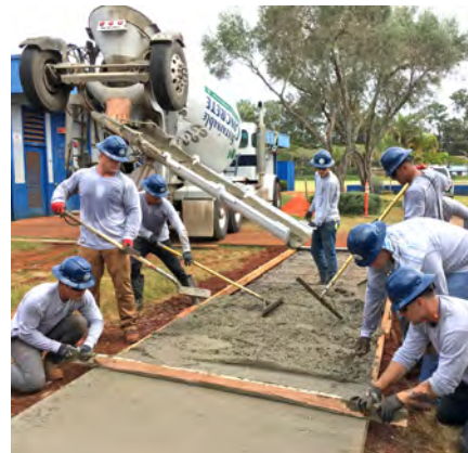
In Progress: Placing concrete
