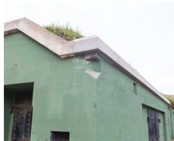
After: Repairs complete
