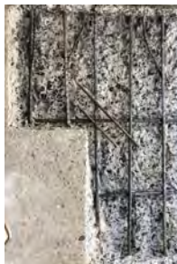
Partial depth slab repair: concrete removal; reinforcing
