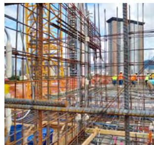
Team field trip to learn about high-rise building construction
