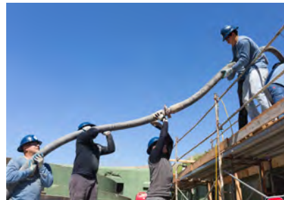
Concrete from ready mix truck delivered through pump and hoses; all hands on deck to manage hoses heavy with concrete
