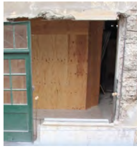
Historic window removed during construction
