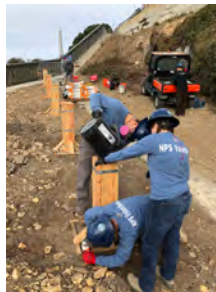
Constructing walkway at base of stairs
