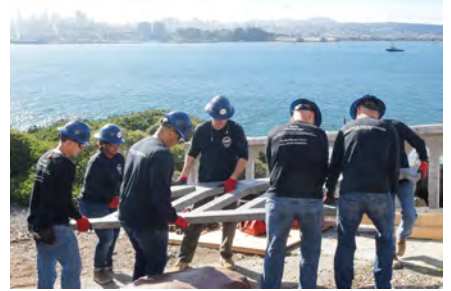
Transporting 300-pound precast concrete panel up hill
