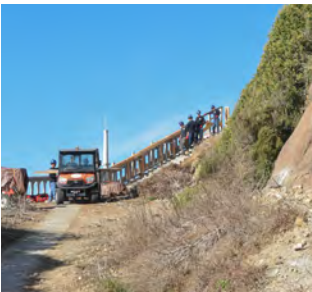
Work site with difficult project access from below
