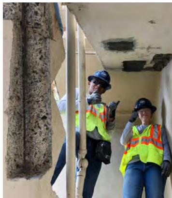
In Progress: column and soffit repairs
