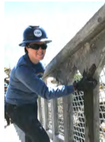
Installing welded wire mesh for visitor safety
