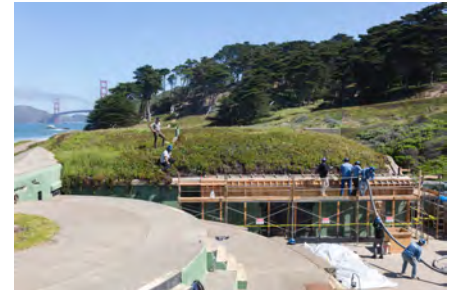
Work site; Golden Gate Bridge in background
