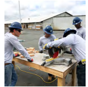
Building custom formwork
