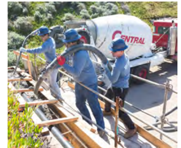
In Progress: concrete placed via pressure pumping
