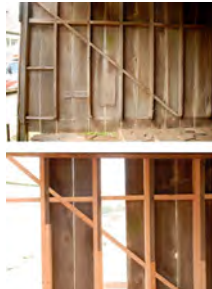
Top: Existing condition; Bottom: preserved/new members
