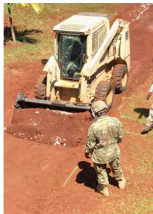
In Progress: Site preparation
