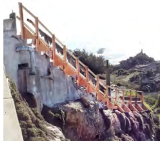
CPI constructed safety railing in place during project
