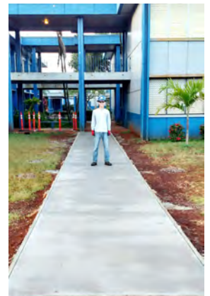
After: Completed project
