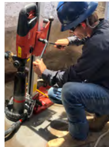
Vertical core drilling for material testing
