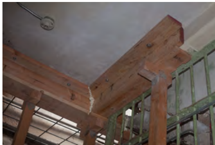
Beam formwork; new beams support repaired landing at top of stairs
