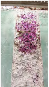
Concrete carbonation testing
