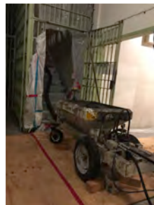
Concrete pump with hoses reaching up into confined space
