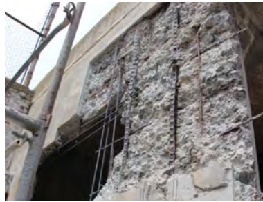
Deteriorated concrete removed, reinforcing steel cleaned/new steel installed
