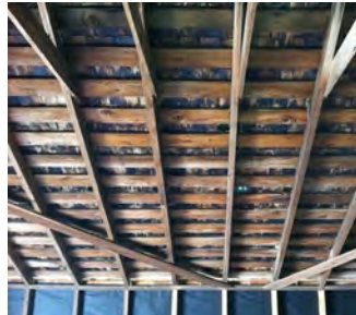
Completed roof interior, preserved historic framing & decking remain visible
