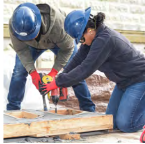
Removing formwork from completed precast panel
