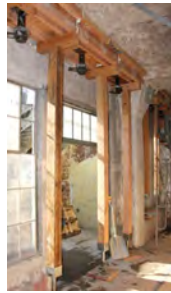
Interior façade beam formwork
