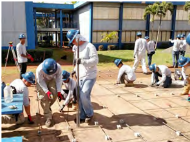
Reinforcing steel placement
