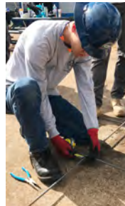
Measuring & cutting reinforcing
