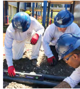
Placing pipe to be embedded in concrete
