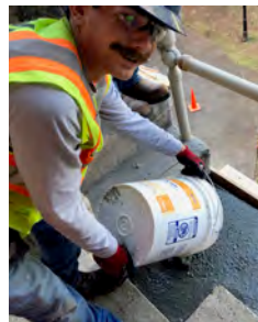
Partial depth slab repair concrete hand placed
