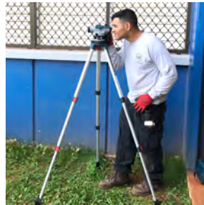
Project planning: site surveying
