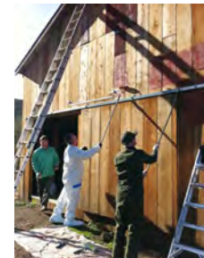
Painting repaired barn with NPS staff
