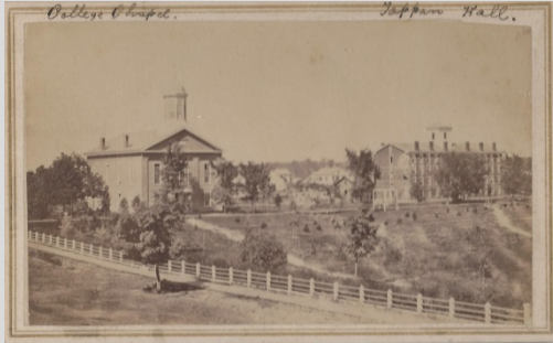
Tappan Hall On The Campus Of Oberlin College
