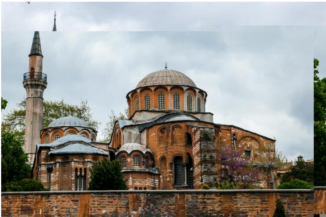
Picture 2: The Church of the Holy Savior in Chora
